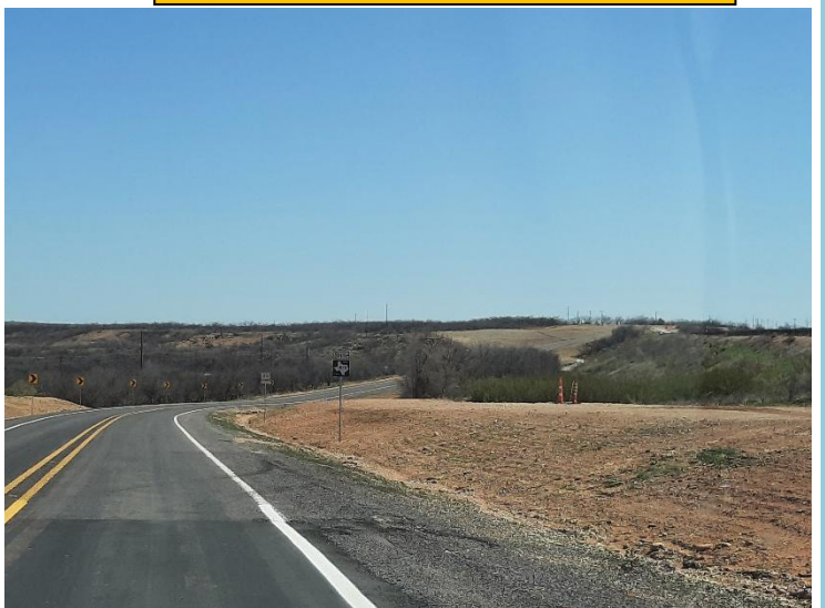
New Roadway FM 1082 (03-24-25)
